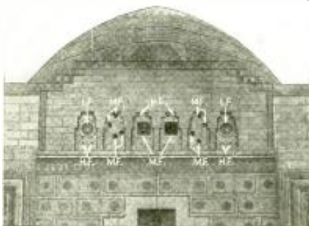
Fig. D A front view of the complete speaker set-up. The "baffle" actually measures about 50 x 70 feet high! About 20 (assorted) reproducers are shown.
