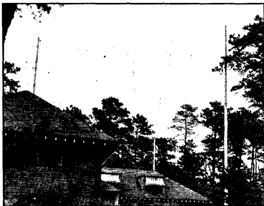
PART OF WICCZ'S ANTENNA SYSTEM
