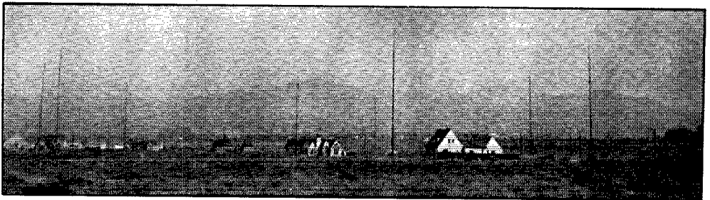
W6GRL really goes in for antennas. The nine tall poles that can be seen all help support the antennas, and there is one more pole that couldn't be squeezed into the picture. One pole is 105 feet high, and the rest are only a measly (by comparison) 70 feet.
