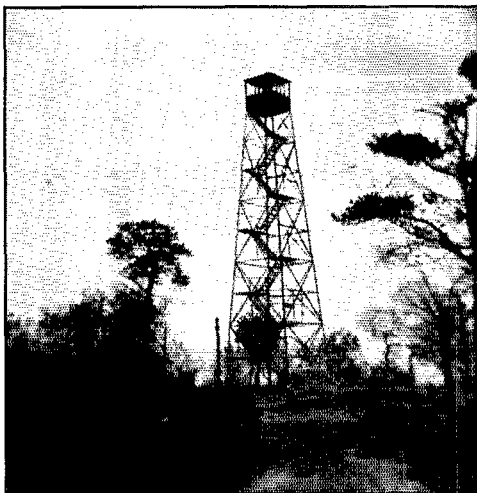
The 65-foot fire tower used to support the di-pole antenna at W8CIR/8, Tuscarora Summit, Pa.
