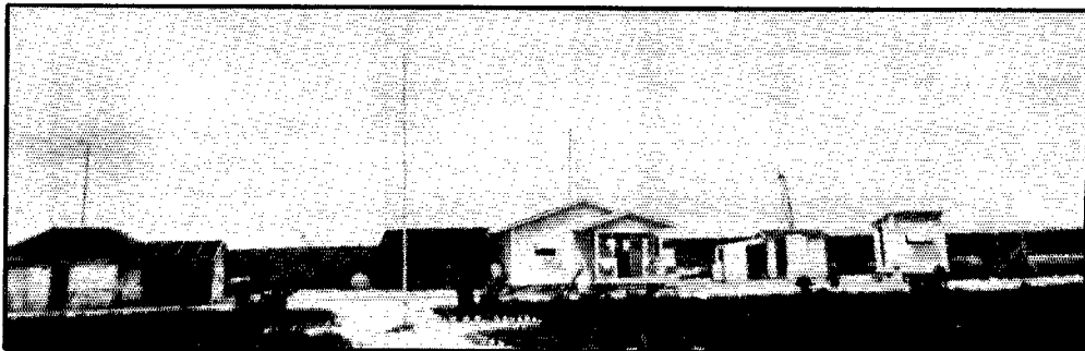
Howland Island is made up of these buildings — and sand! From left to right: kitchen and food storage house, rain collection shed, government house (sleeping quarters and radio station), tool room and generator house, and hydrogen shack.
