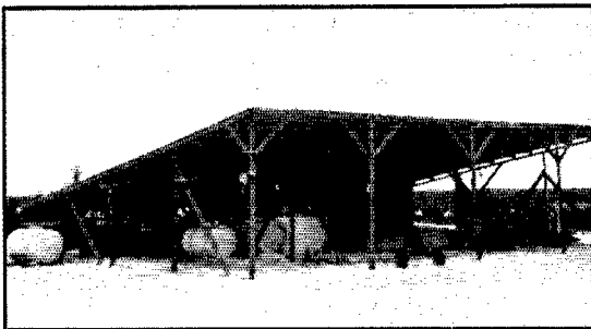
Drinking water was collected on the roof of this shed and fed into drums through a trough.
