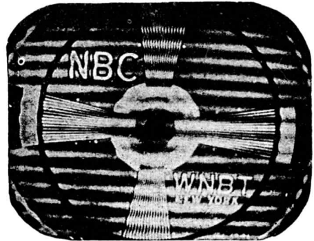
Figure 3-3—Test Pattern Tuning Misadjusted
